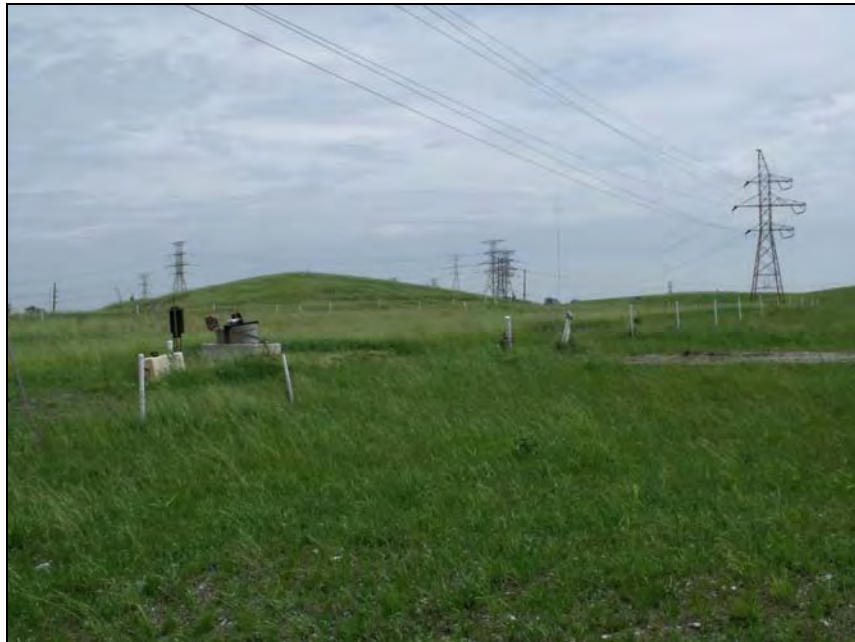
Photo 10: SWMU 1 – regraded cap area
