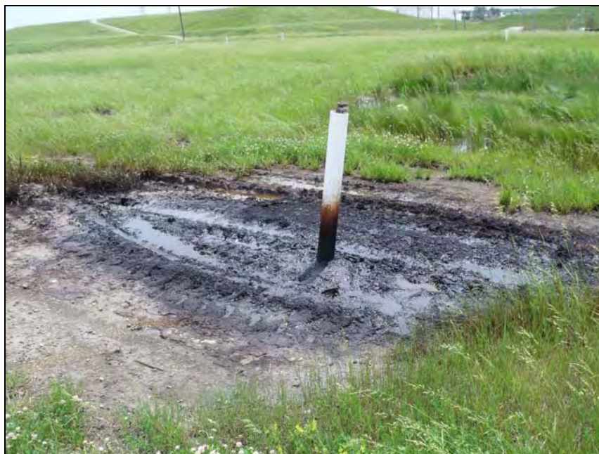
Photo 22: SWMU 9 – stained vent pipe.
