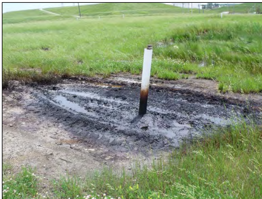
Photo 22: SWMU 9 – stained vent pipe.
